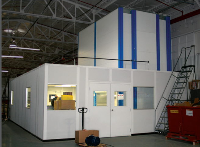
Environmental controlled enclosure to insure production quality
