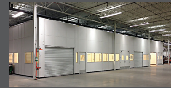
Automotive work bays control fumes & temperature
