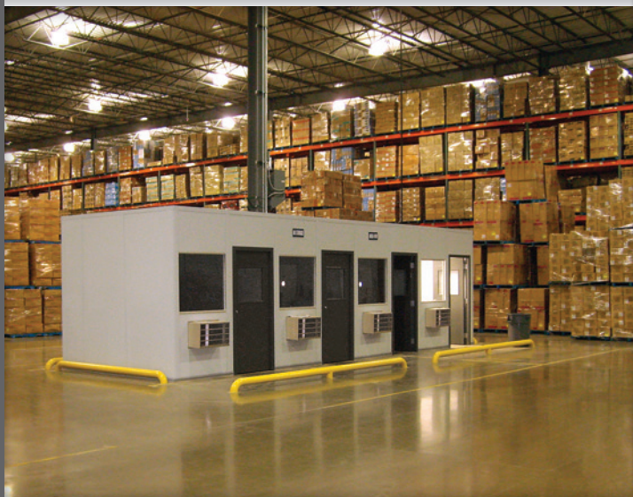
Four, warehouse management offices; constructed of InPlant's Standard Steel System & 3" Painted Gypsum Faced Wall Panels
