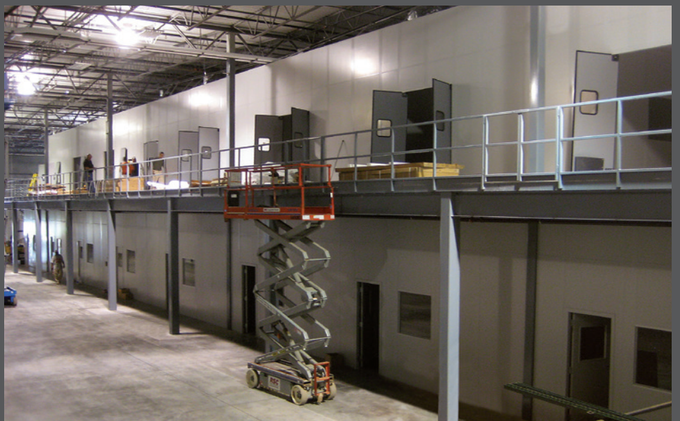
Warehouse storage over lower production rooms, 3' 16 gauge Heavy-Duty Steel System & tall Wall Panels
