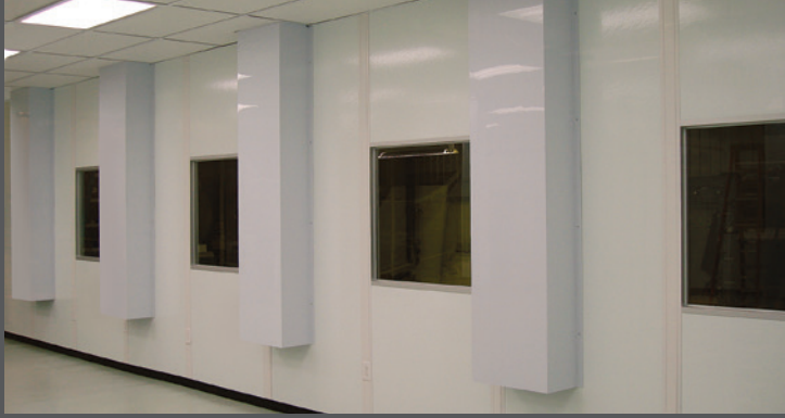
Designed to support equipment that regulates temperature and humidity
