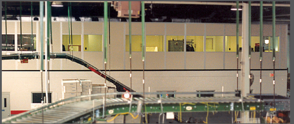
Modular Light-Weight Aluminum System, administrative offices erected over existing production rooms
