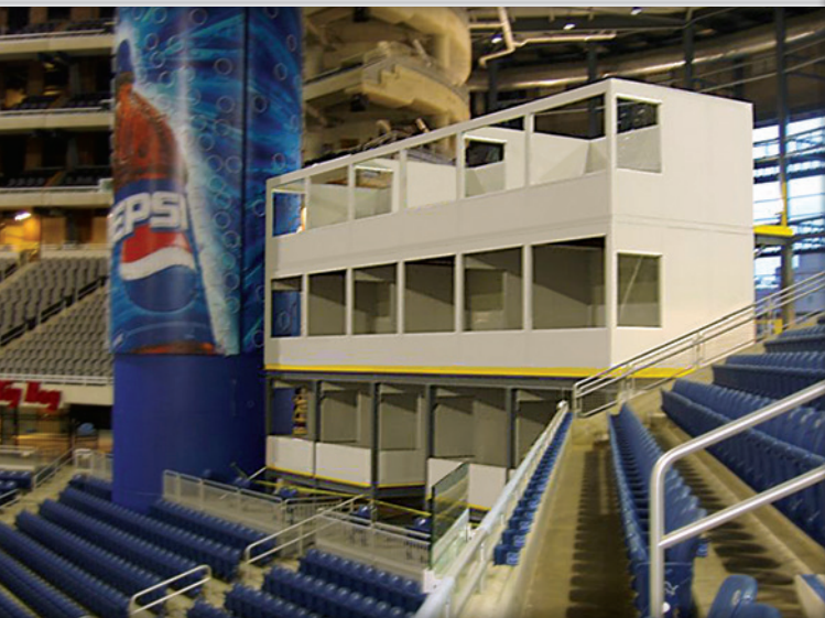
Partitioned suites on a mezzanine for media coverage; constructed of InPlant's Versatile Steel System & 1 3/4" Painted Gypsum Wall Panels
