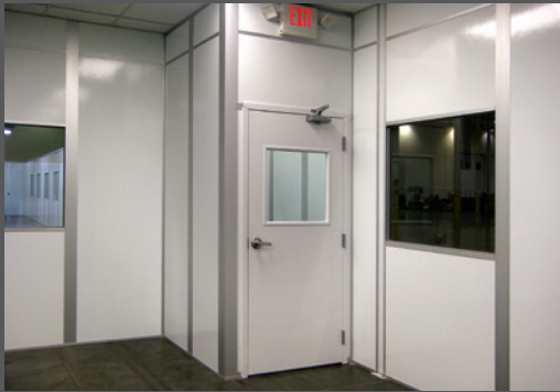
Temperature & contaminant controlling entrance, 1 3 / 4 " Light-Weight Aluminum System & FRP Faced Wall Panels
