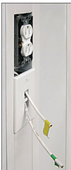
The Cover Plates in the Wiring Studs are cut to open sections for outlets and switches.
