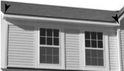
Measure the length of the trim piece. Be sure to add for corner or end laps. If trim piece length exceeds the length of the brake, measure for two pieces and determine best point for overlap.
