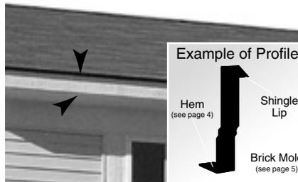
Measure the width of the trim piece and where each bend will be made. Tech tip: Use a small strip of the material and hand bend it into a profile of the area your trimming off. You can also use the "profile" to check the rest of the job where the same trim piece is to be used.
