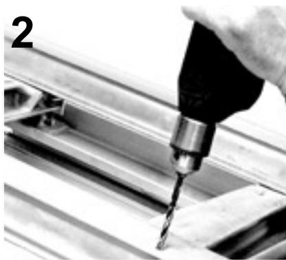
After repeating step 1 on opposite base rail, use bit in parts bag to drill all four holes. Use center punch if needed.
