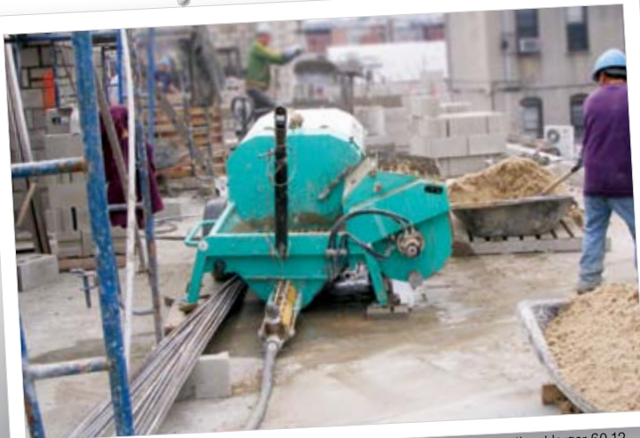
Concrete block walls are being filled with the Silent 300 which is shown with the optional larger 60.12 rotor/stator. Notice the grout is being made the old timey way – shovels of sand and some portland.
